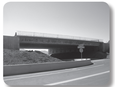
Parker Ranch Road Grade Separation and Kelly Canyon Road.
