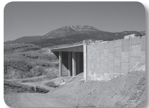
Browns Creek Bridge.
