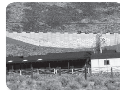
Mechanically Stabilized Earth (MSE) retaining walls.
