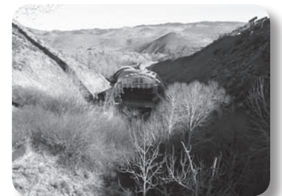
View of the temporary arch culvert that spans Galena Creek. Fill material approximately 100 feet high will be placed on top of this culvert to assist in the construction of the Galena Creek Bridge.
