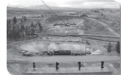
Foundation construction at Galena Forest Bridge.
