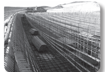
Steamboat Hills Bridge superstructure (soffit and stem walls) under construction.
