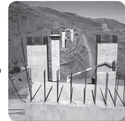
Northern view of bridge piers at Galena Creek Bridge.
