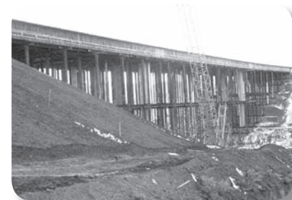
Steamboat Hills Bridge with completed falsework.
