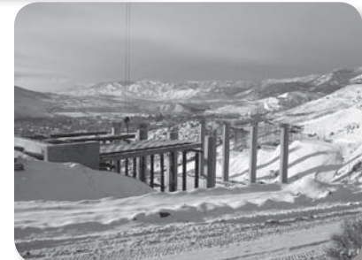
View of Pleasant Valley Bridge during falsework assembly.
