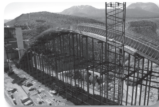
Galena Creek Bridge southbound arch falsework construction.
