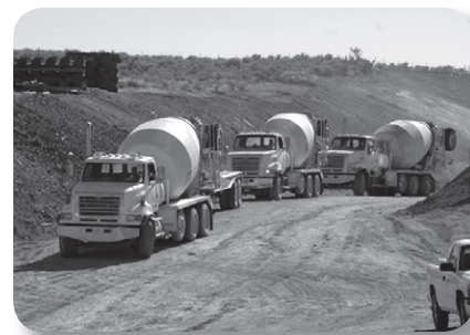
Convoy of concrete trucks traveling through the project site.
