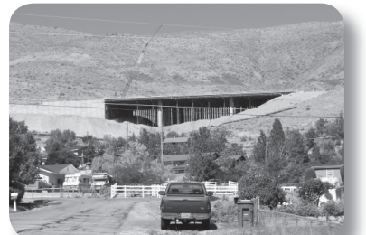
Pleasant Valley Bridge looking west from surrounding neighborhood.
